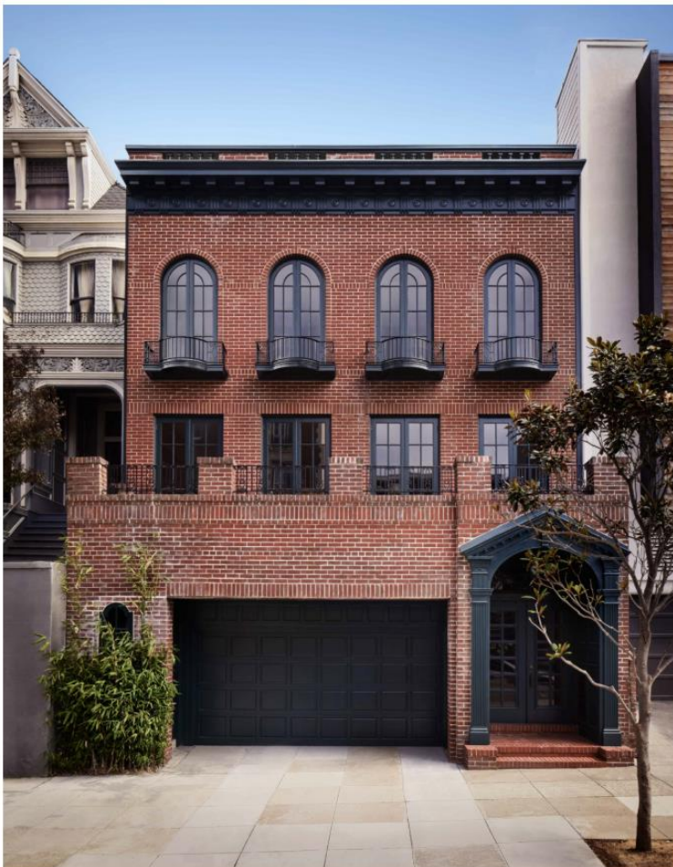
ABOVE The arched doorway and windows at the front façade were preserved while the trim was repainted
